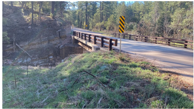
Photo 1 Colcord Road bridge
