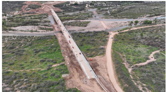
Photo 2 Tonto Creek bridge (in progress)
